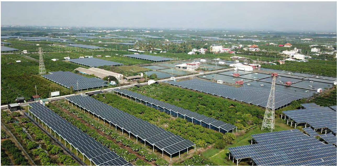
Figure 3 – Solar power generation in land subsidence area
